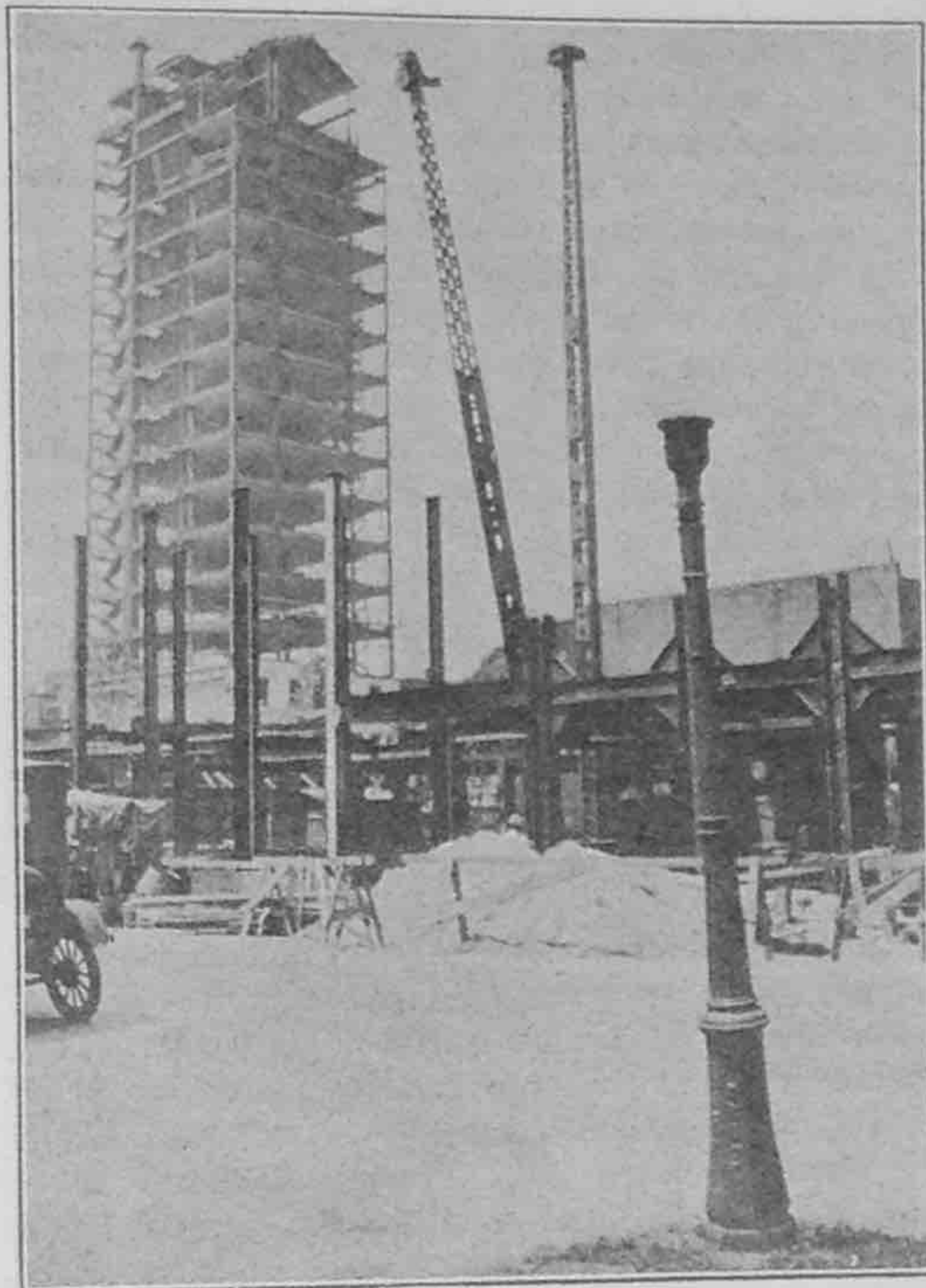
BUILDING A CHICAGO SKYSCRAPER
